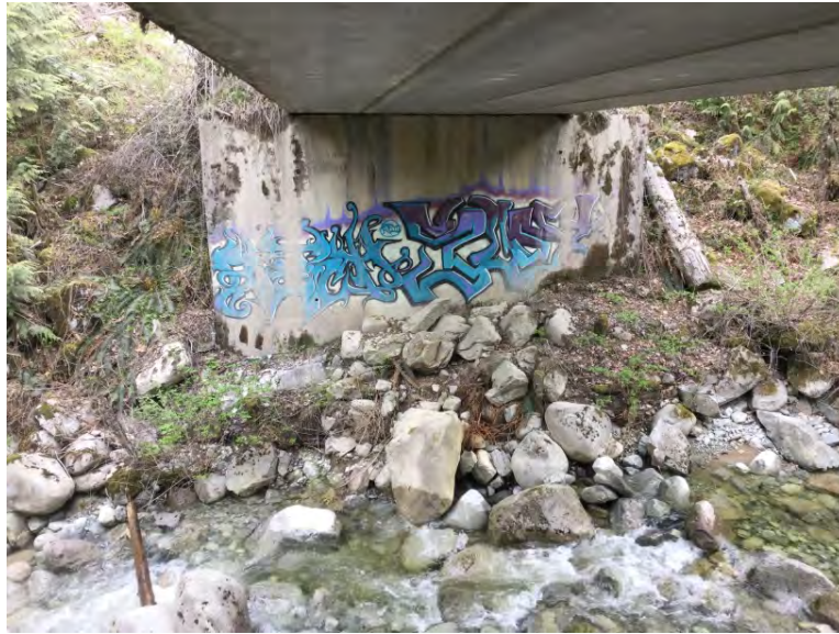
Right Bank Abutment when facing downstream
