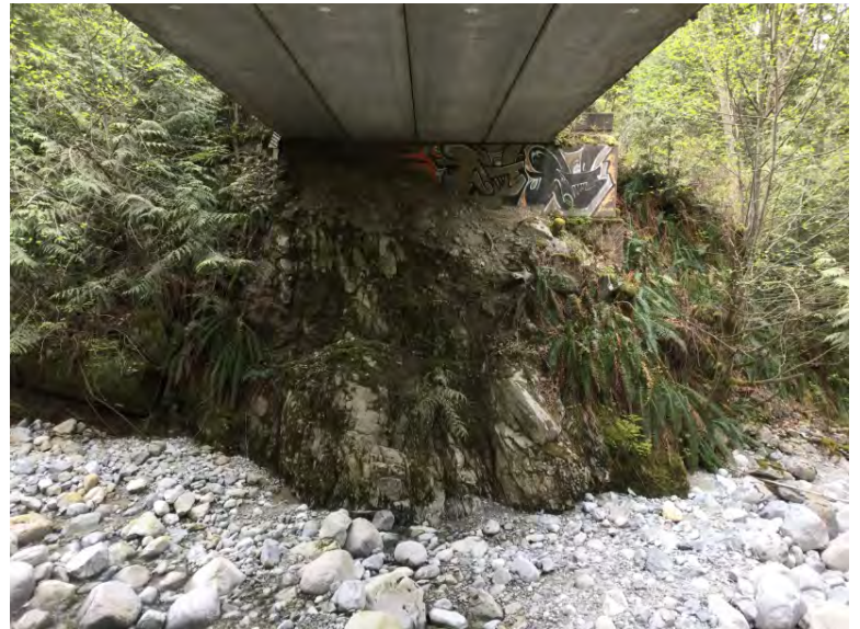
Left Bank Abutment when facing downstream
